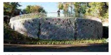
A 0.9 million above-ground stormwater storage tank with an art wall. Madison Valley Stormwater Project Phase II, Seattle Public Utilities
